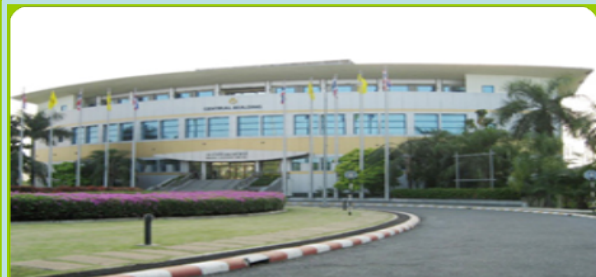
PTT, Wangnoi & Rayong Model: BYZ233 Fuel: Direct Fired (NG) Cooling capacity: 750RT x 5 sets
