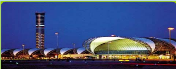
Suwannahumi Airport TRI-GENERATION SYSTEM (Gas Turbine + HRSG + Absorption Chiller) steam Model: BS600 Cooling capacity: 2500RT x 4 sets
