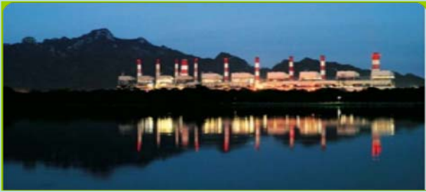
EGAT – Mae Moh Power Plant , Lampang Blowdown Heat Recovery to Air-conditioning System Model: BS125 , BS150 Cooling capacity: 1,150 RT
