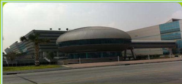
New Thailand Government Center Fuel: Exhaust Gas from Gas Turbine 5 MW x 2 Model: BE1000 Cooling capacity: 3,300RT x 2 sets
